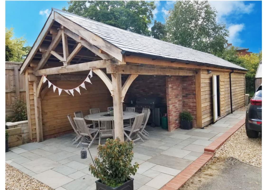
Primary structure of green oak frame consisting of 6 posts with 3 king post trusses over and high level perimeter beams all around. Additional structure in single brick forming Bike / BBQ store rising above ridge as capped tower construction. Trusses support 6 purlins running full length of building plus eaves.
